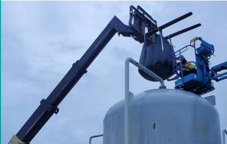
Contractor Filling Media Into GAC Tanks
