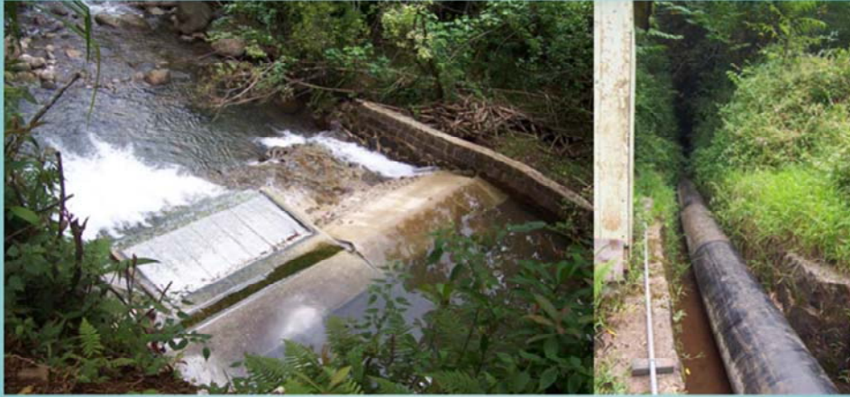
Renovated Punalu‘u Stream Diversion
