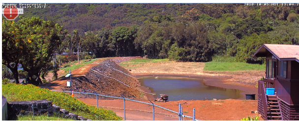
Photos: Before and After Pumping
