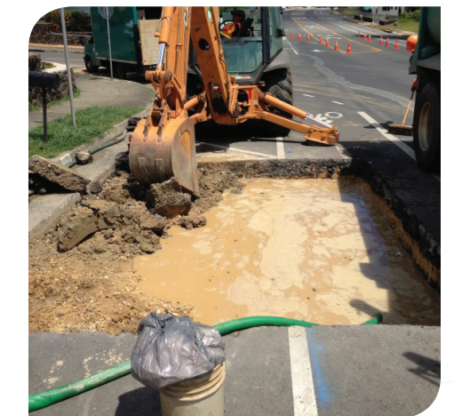
The BWS's crews must remove water from a trench during excavation
