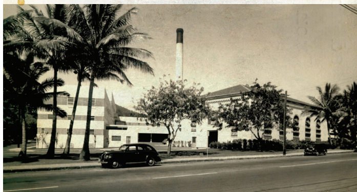
The Beretania pumping station circa 1940.
