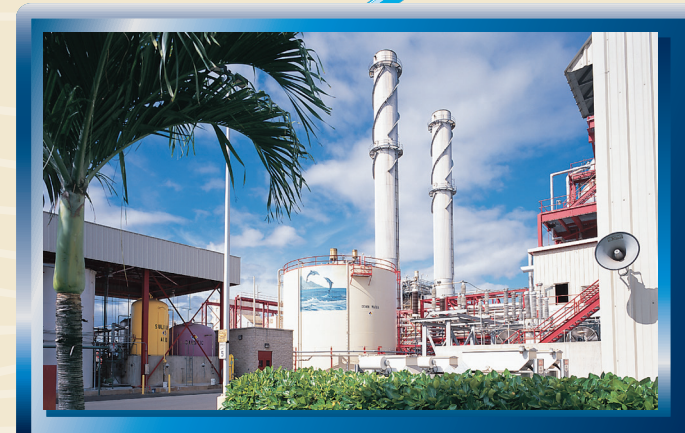
RO water is used for industrial cleaning or to make steam for oil processing.
