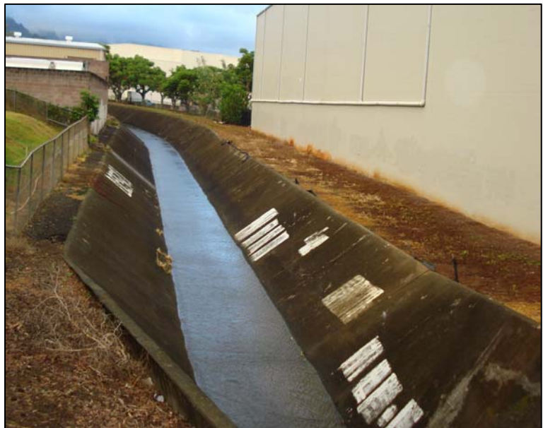
Kahuhipa Street storm drain
