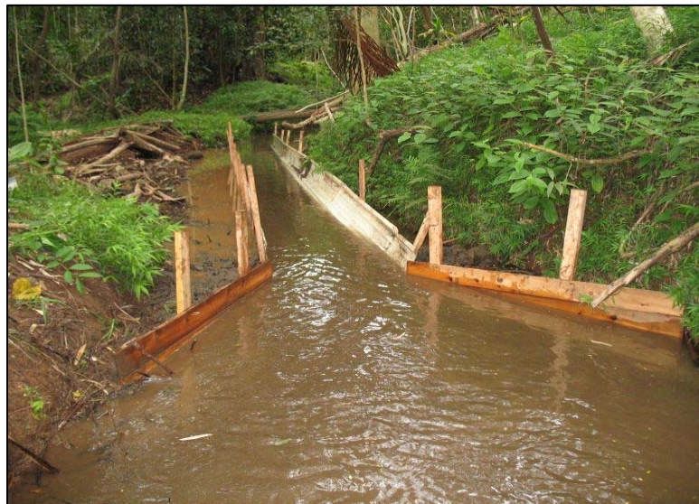
Temporary upgrades of the Waimānalo Irrigation System
