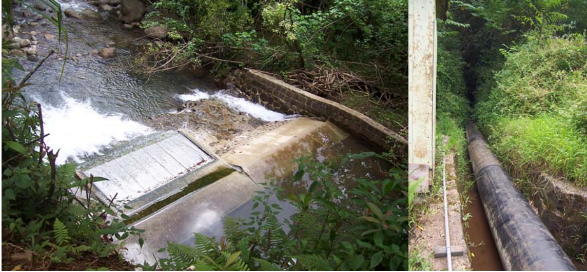
Figure 1.6 Punalu'u Stream Diversion and Piped Ditch
