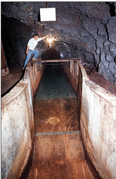
Waiāhole Ditch, north portal Photo credit: George F. Lee Star-Bulletin, April 25, 1997
